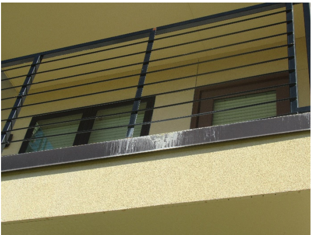
Stain at balcony flashing
