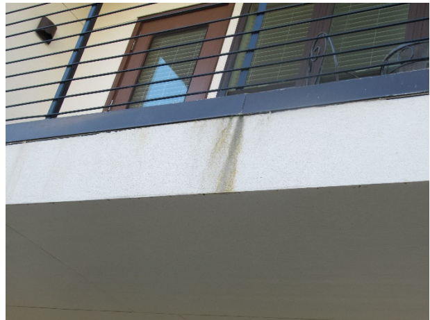
Staining at stucco finish
