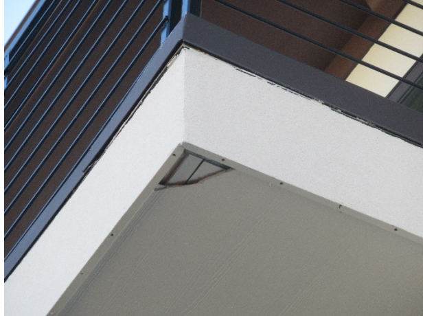
Damaged soffit
