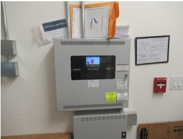
Fire control panel and emergency device
