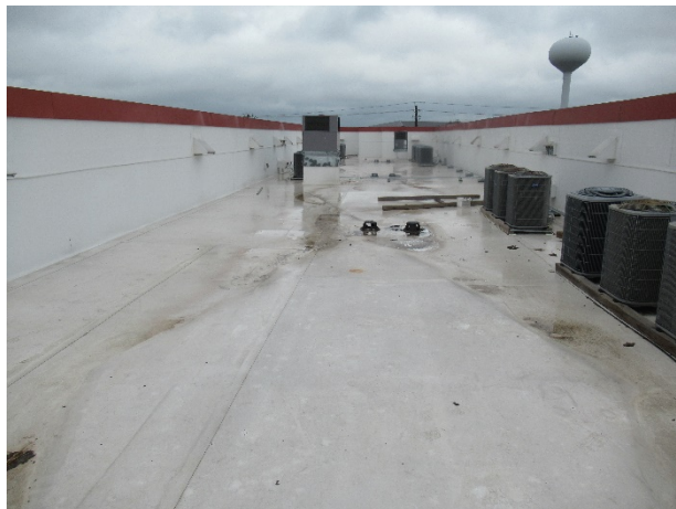
Discoloration at roof
