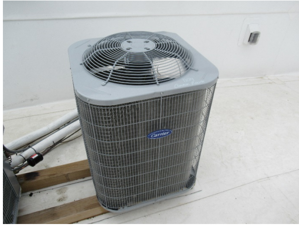
External condensing unit
