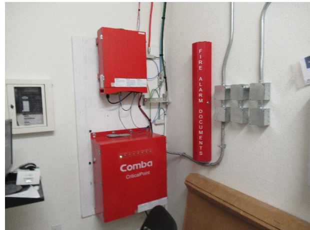
Emergency radio signal booster panels
