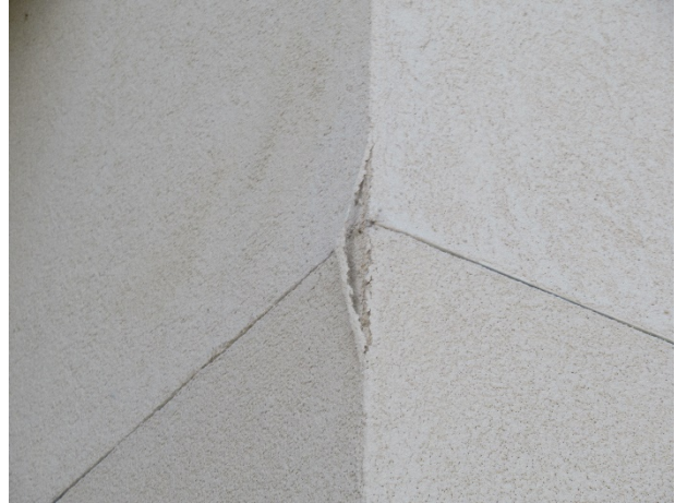
Minor stucco damage
