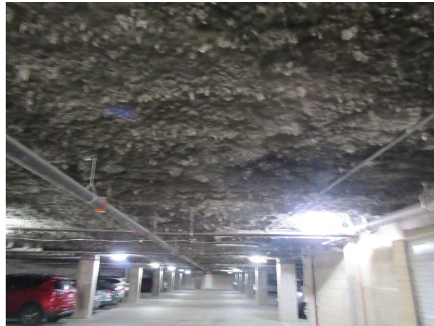
Spray foam insulation at the garage
