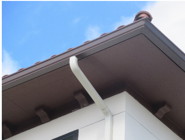
Gutter and downspout assembly
