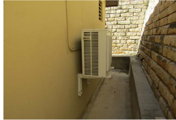
Mitsubishi 1.5 ton air conditioning condensing unit
