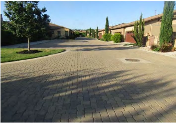
ashlar pattern dry set masonry pavers
