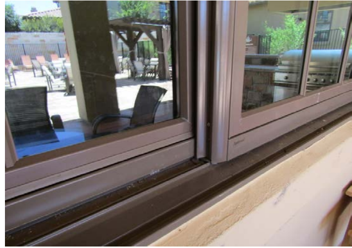
wood frame with aluminum cladding, dual pane glass, sliding window
