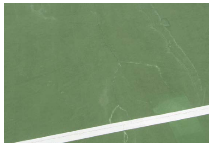
minor cracks
