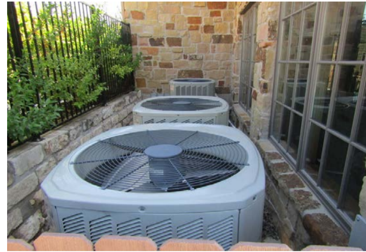
Trane air conditioning condensing units
