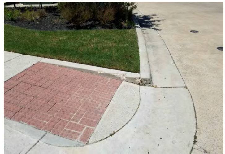
concrete deterioration
