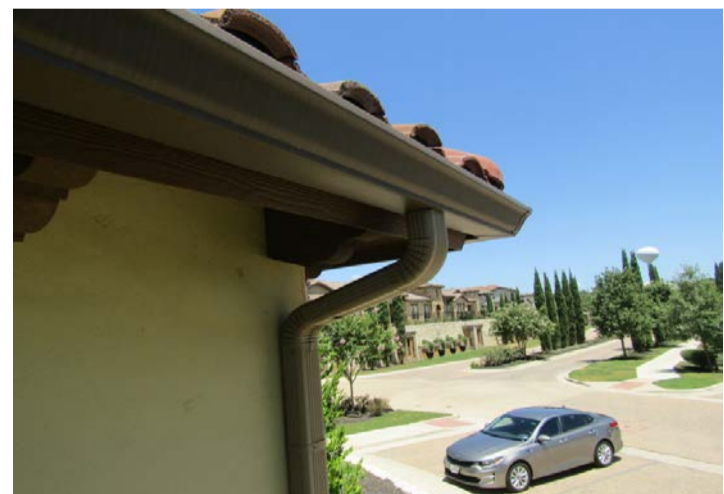
aluminum gutter and downspout
