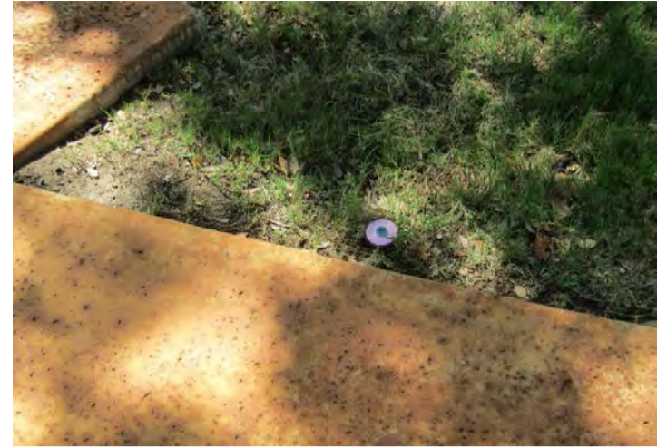
irrigation system head
