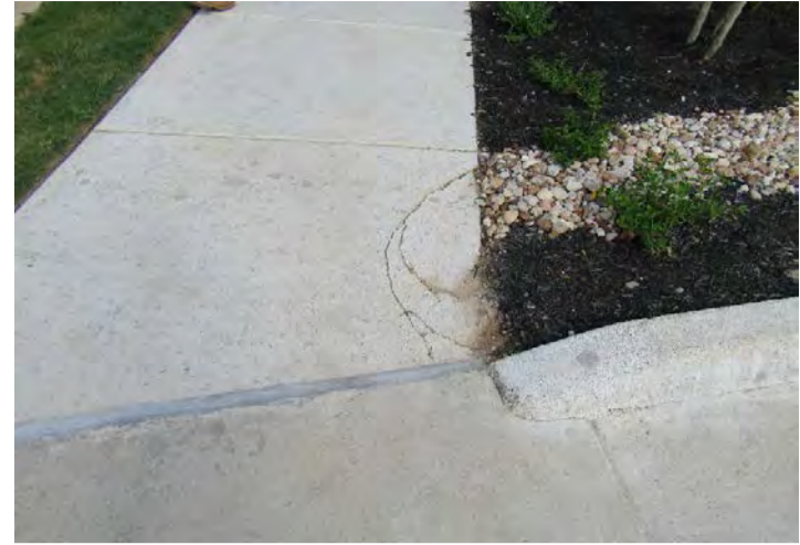
cracked concrete
