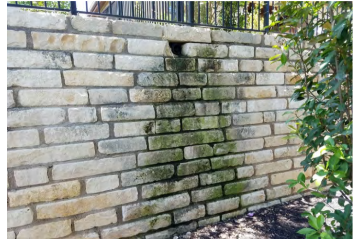
water stains - consider installing piping to direct water down the wall and discharge 10 feet from the wall base
