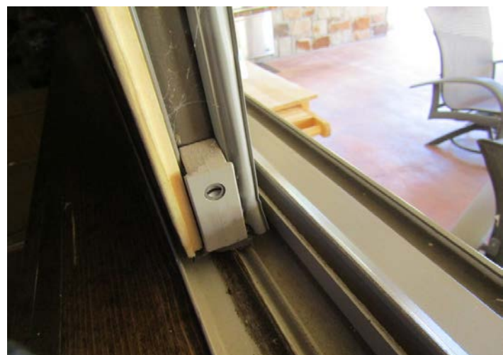
sliding window with bulb-type weatherstripping
