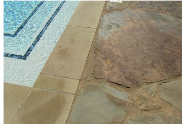
joint not caulked between tile and deck
