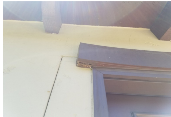
trim deterioration
