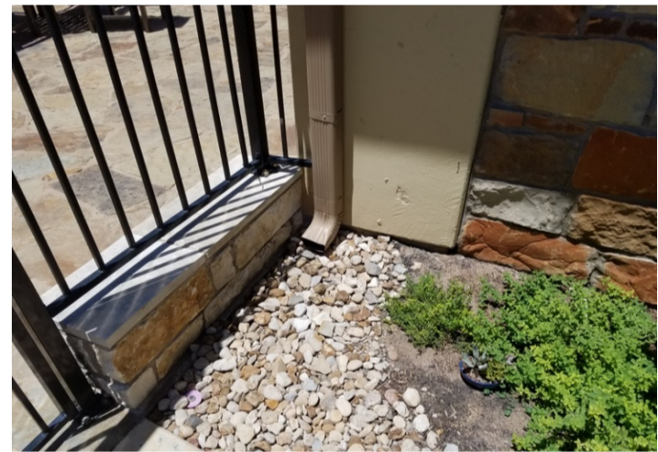
discharge at foundation
