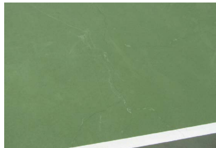
minor cracks
