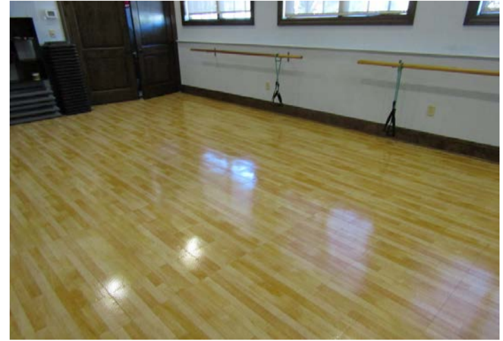
vinyl flooring in the yoga room with wood trim transition at floor to wall
