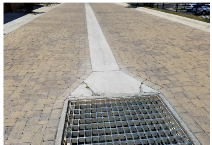
damaged concrete
