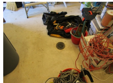
Figure 1: Floor drain higher than the floor in the large clubhouse storage room
