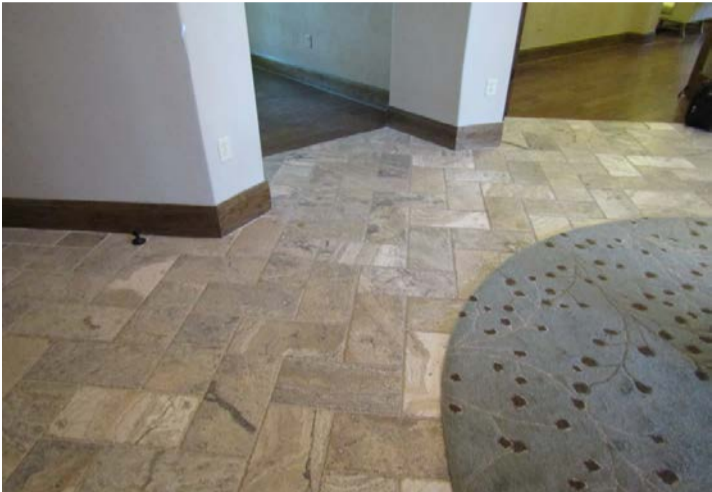
16 inch by 8 inch tile with wood trim transition at floor to wall
