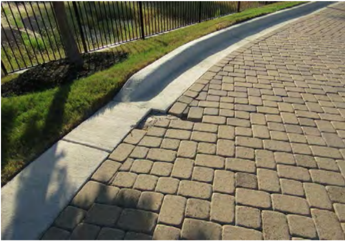
missing/damaged pavers at townhomes
