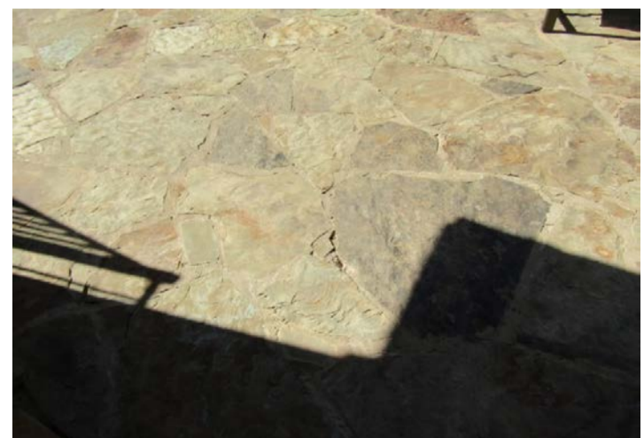
mortar deterioration
