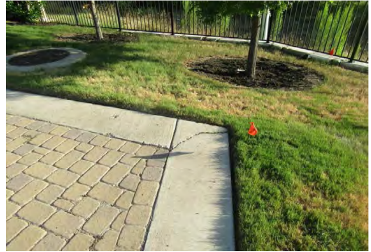
crack in concrete
