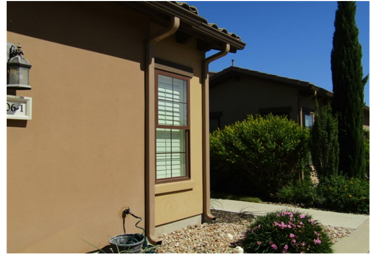
aluminum gutters and downspouts
