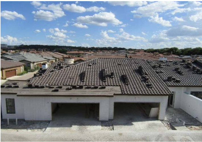
roof tile placement
