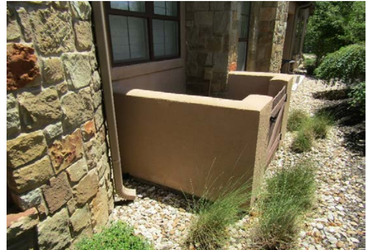
downspout discharges too close to foundation
