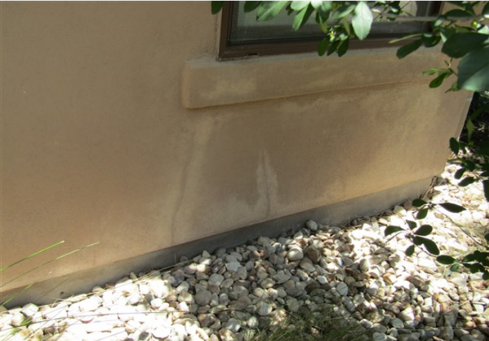
cracks in stucco
