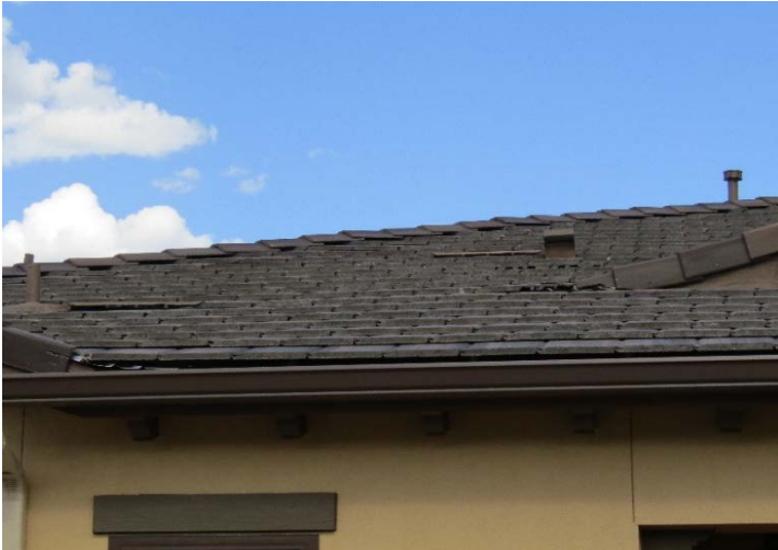
tile roof with penetrations
