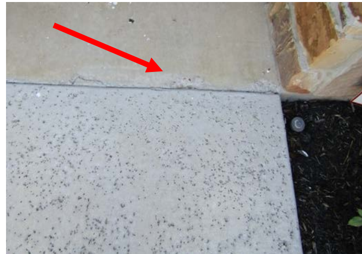
minor cracks and spalls - no action necessary
