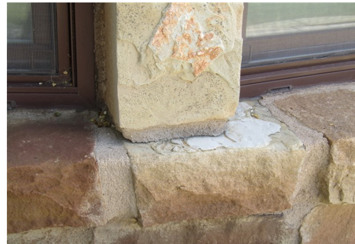
minor mortar deterioration is evident
