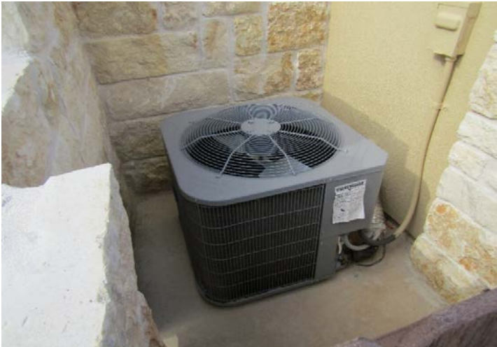
concrete air conditioning (A/C) pad
