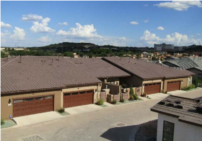
roofs with concrete tiles
