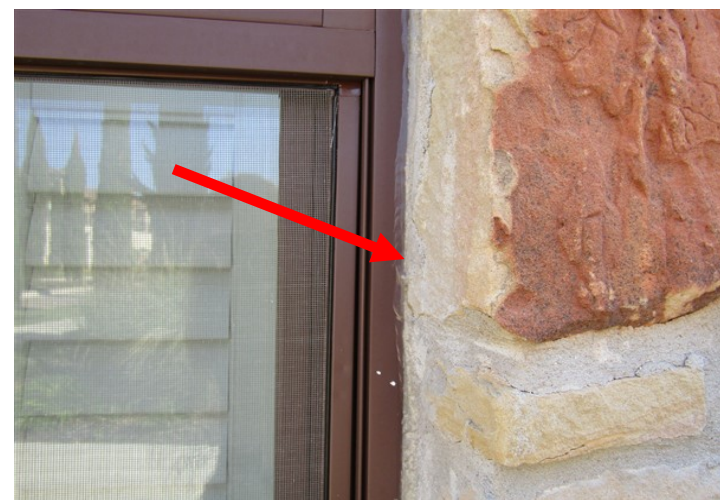
caulk at window and masonry
