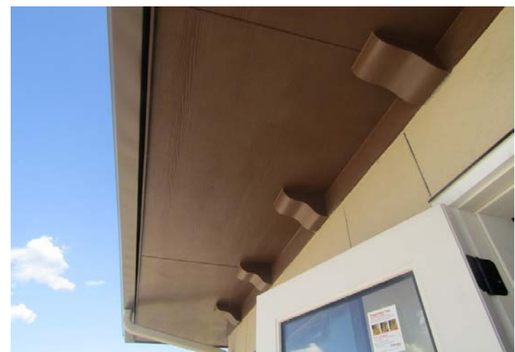
paint at soffit, fascia and frieze board
