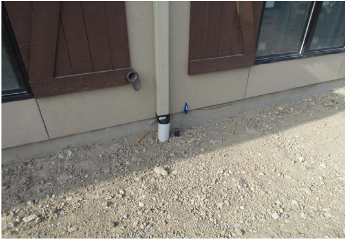
downspout connected to subterranean piping
