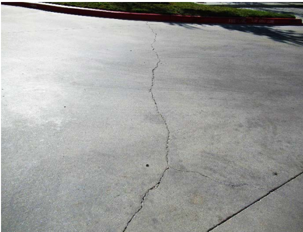
Concrete cracks at the parking area
