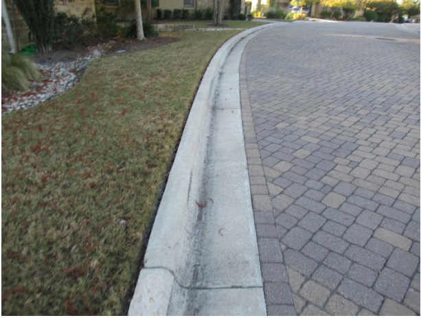
Concrete curb and gutter
