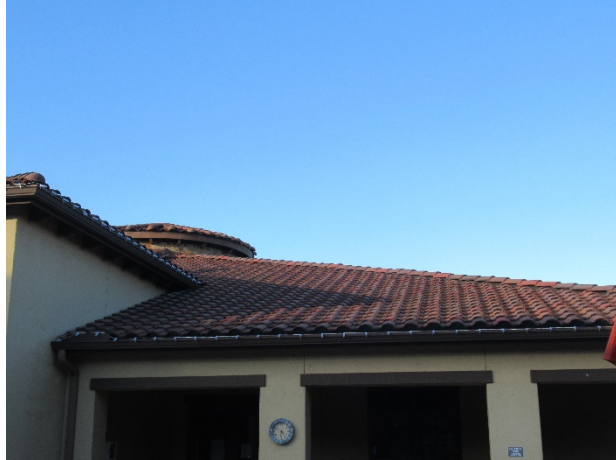
Concrete tile roof overview
