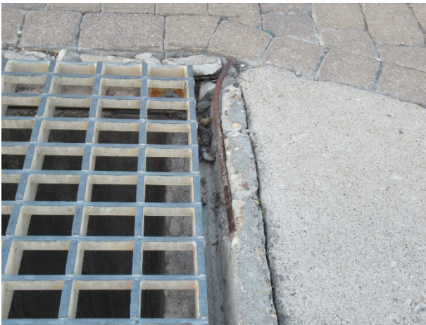
Damaged concrete and exposed reinforcement steel
