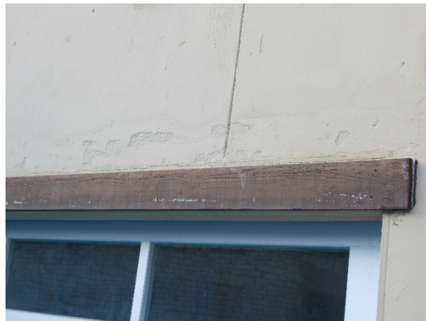
Minor finish deterioration at wood trim
