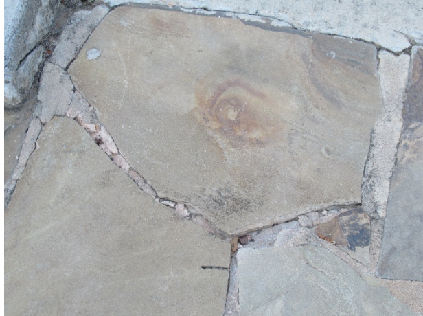
Mortar deterioration
