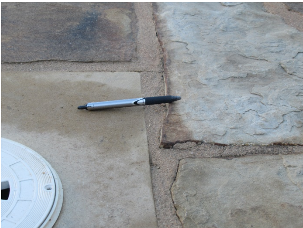
Trip hazard due to settlement
