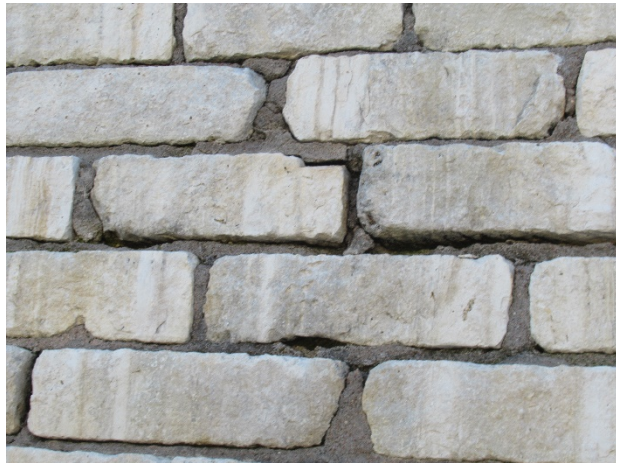
Mortar deterioration
