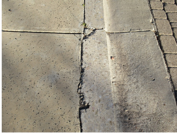
Concrete damage at curb
