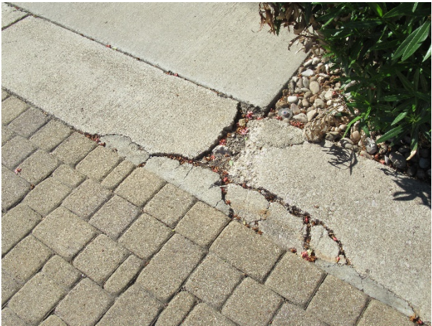
Concrete damage at curb
