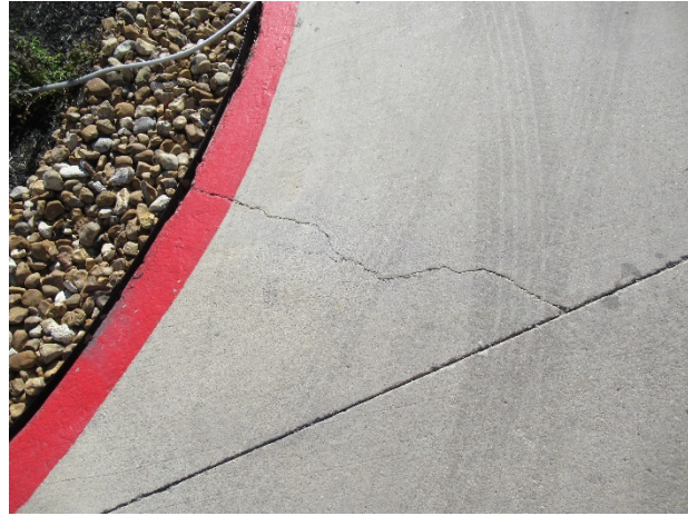
Concrete cracks at the parking area
