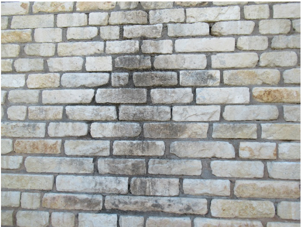
Discoloration and mortar deterioration
