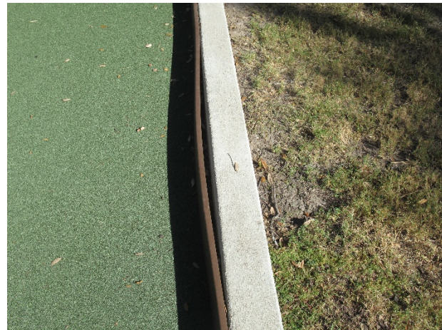
Warped timber border
