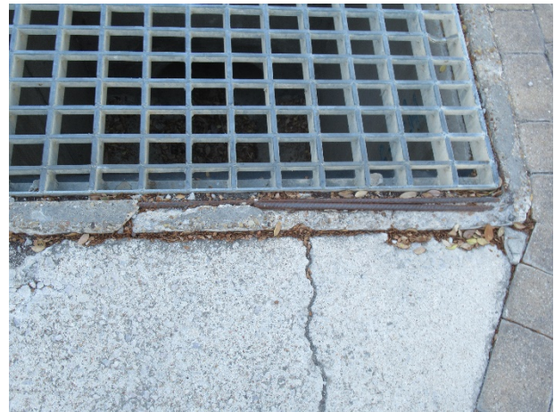
Damaged concrete and exposed reinforcement steel
