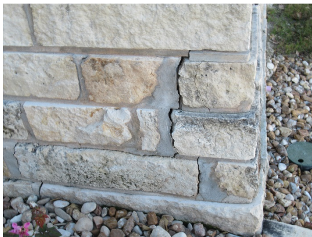
Mortar cracks
