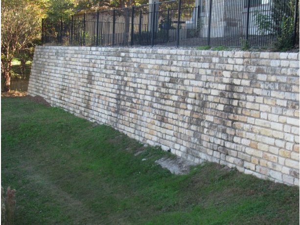
Masonry retaining wall overview – Note discoloration
