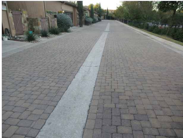
Concrete gutter
