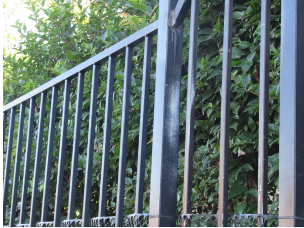
Finish deterioration and minor rust
