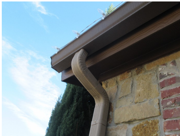
Gutter and downspout assembly
