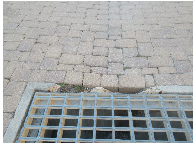
Concrete damage around the catch basin – Note sunken pavers
